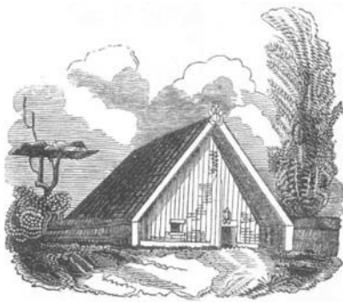
Native house erected for a European,
