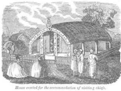
House erected for the accommodation of visiting chiefs,
